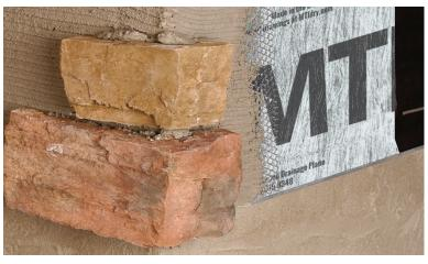
Thin Stone with Sure Cavity rainscreen drainage plane
